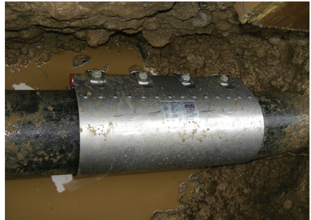
Repair of large damaged areas up to 250 mm
