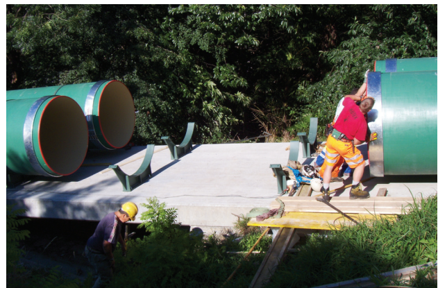
For the installation of an adapter piece
