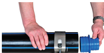
Push the reducer into the first tube until it stops
