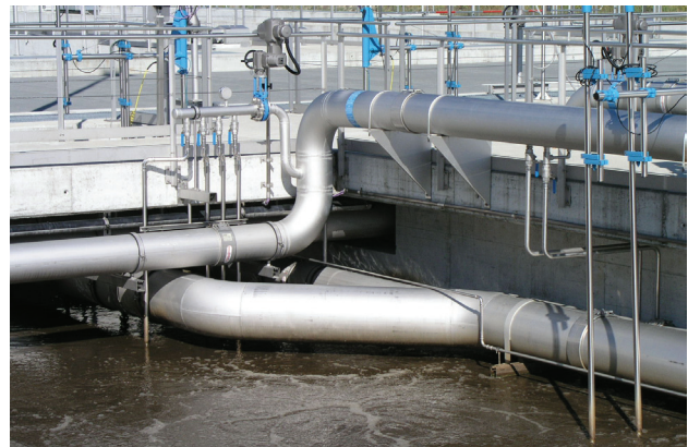
Prefabricated pipe section are installed with STRAUB-GRIP-L
