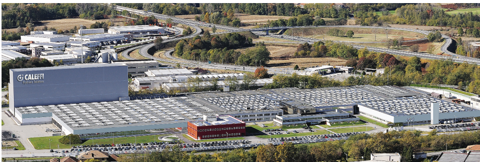
Caleffi S.p.A. - Corporate Headquarters - Plant 1 Fontaneto d'Agogna - ITALY
