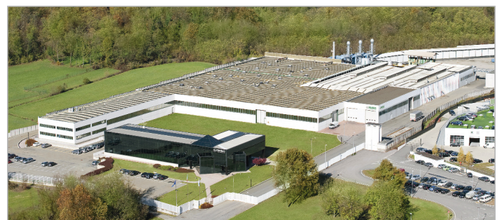
PRESSCO S.p.A. - Hot pressing and mechanical processing of brass components Invorio - ITALY
