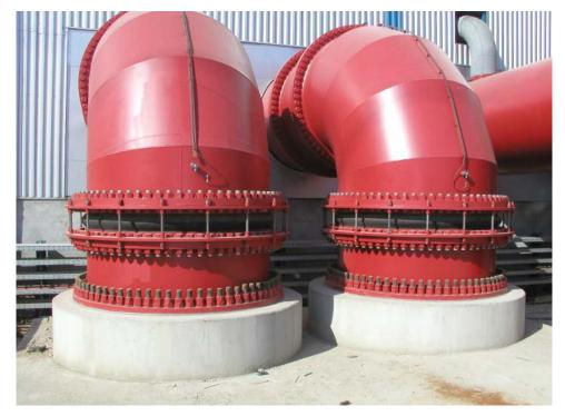
restraint compensator - design M DN 2600
