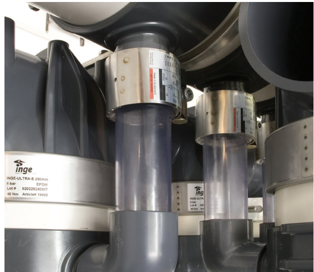
STRAUB-ECO-GRIP is suitable for the connection of sight glasses
